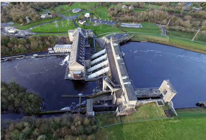
Ardnacrusa Hydroelectric Station, Ireland
