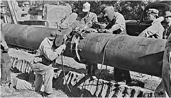
Workers assembling sections of the Big Inch Pipeline.
